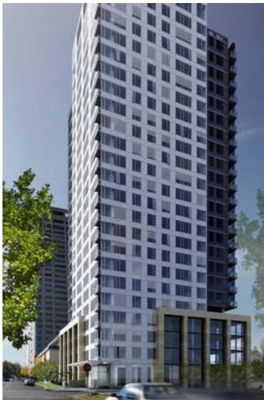
A rendering of 1321 Seneca, a planned 24-story condo tower in Seattle's First Hill neighborhood, an area being marketed in Asia as student friendly. Weber Thompson
